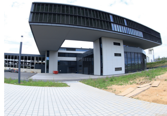
TOWERING STORIES ABOVE THE GROUND, THE OPEN-CONCEPT PLAN CONSOLIDATES STAFF FROM SEVERAL OTHER BUILDINGS, ENABLING INCREASED COLLABORATION AND INTERACTION.
